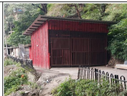
Picture 3.32: Common BM waste collection center at IGMC, Shimla.
