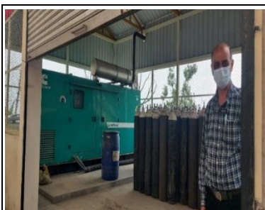
Picture 3.48: Civil work with DG set
