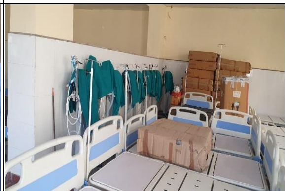
Picture 3.14: Uninstalled and idle equipment of Trauma Centre at RPGMC, Kangra.
