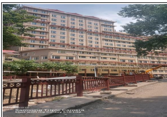
Picture 3.7: Newly constructed OPD block at IGMC, Shimla.
