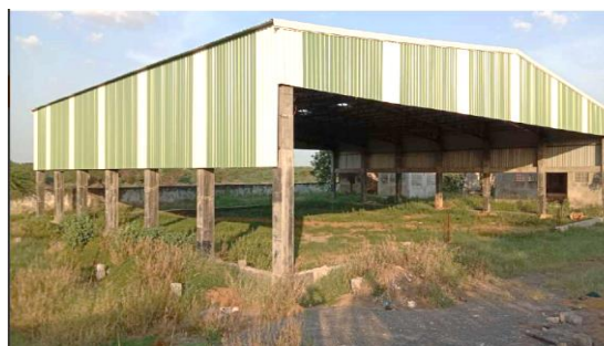
Image 2.24: Status of GTS construction in Ongole Municipal Corporation
