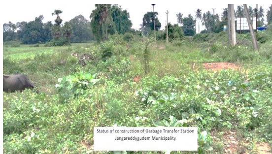
Image 2.23: Status of GTS construction in Janagareddygudem Municipality
