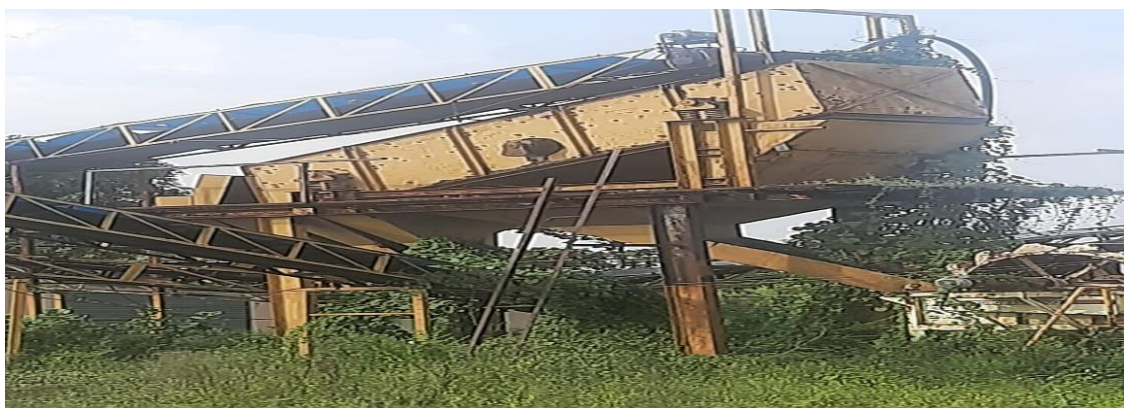
Image 2.27: Non-functioning & Dilapidated C&D plant at Vijayawada
