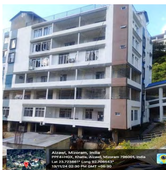
Rear view of the Directorate office building, LAD showing the basements
