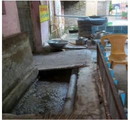
Blocked open drain, passing through the kitchen and washing area for utensils, at DHH, Bhadrak (30 May 2022)
