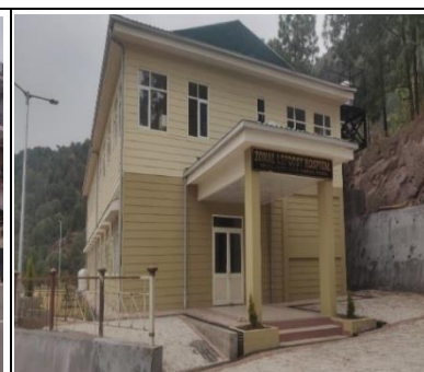
Picture 9.7: New incomplete leprosy hospital at Lohanji
