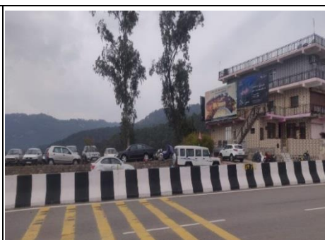
Picture 9.6: Dismantled CHC beside the highway
