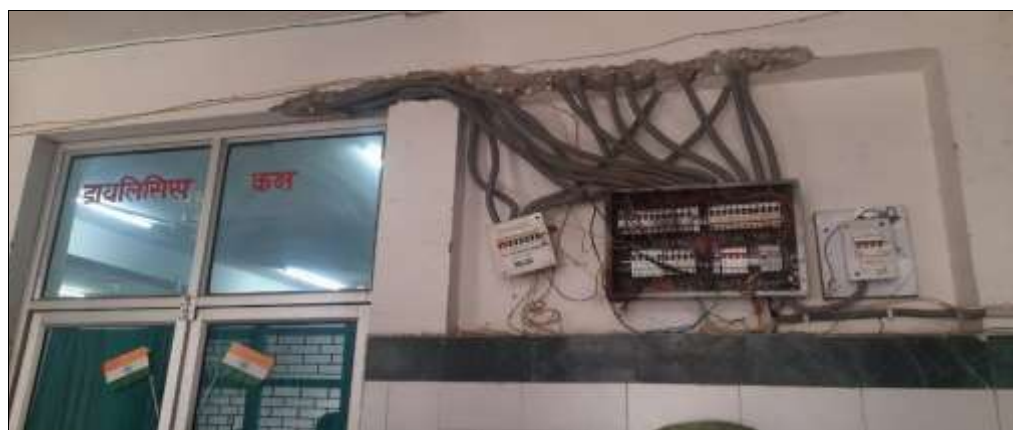
10. Open MCB box in GMCH Bilaspur in risk of short circuit (Date 26 April 2022)
