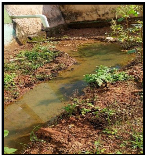
Photograph 3.1.10: Accumulation of waste water, due to lack of any drainage system, at the STGH, KC Pur, Guma Block, Gajapati District
