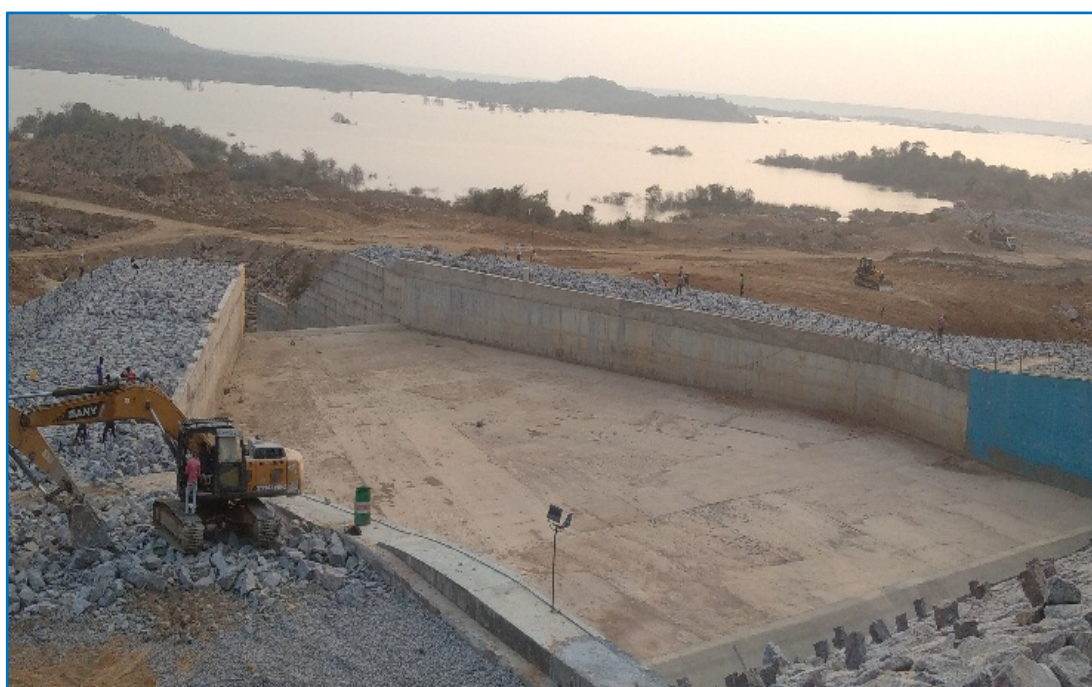
Figure 4.3 - Construction of Ogee Weir on SKMS Reservoir
