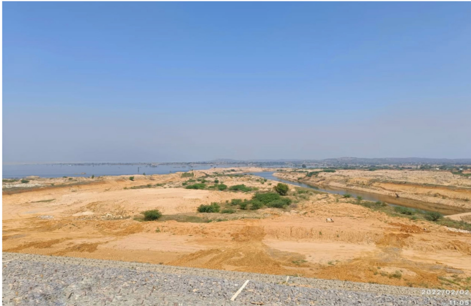
Figure 4.4 - Submerged Feeder Channel inside SKMS Reservoir
