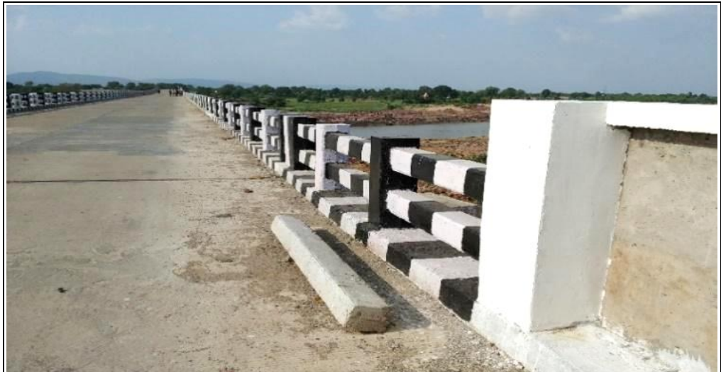
High Level Bridge on Awalihat to Salkanpur Road, Sehore without footpath
