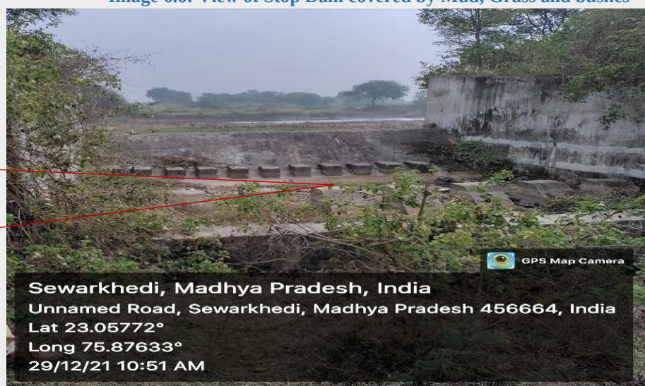
Image 6.6: View of Stop Dam covered by Mud, Grass and bushes
