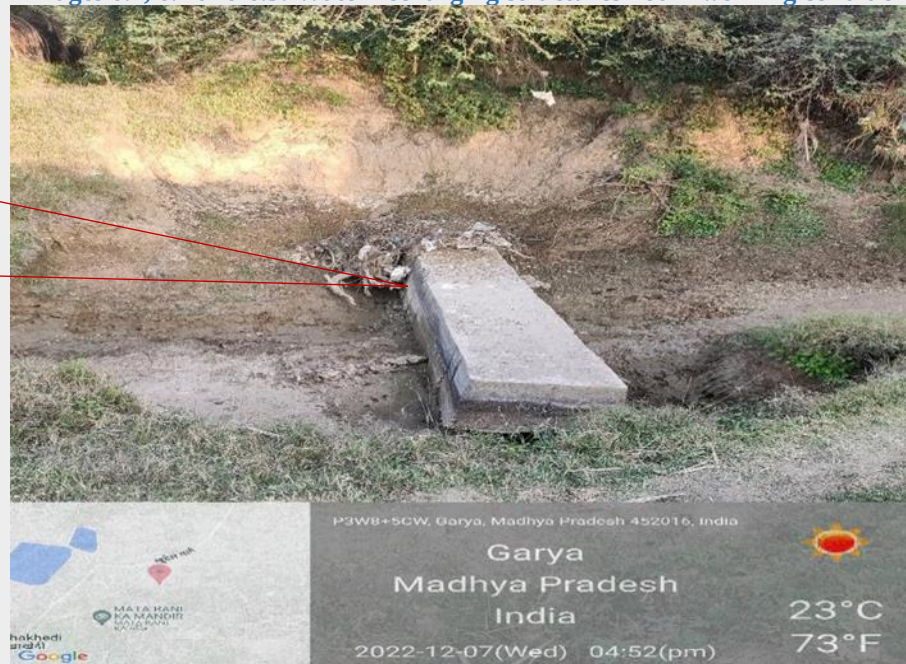
Images 6.1, 6.2 and 6.3: Water recharging structures not in working condition
