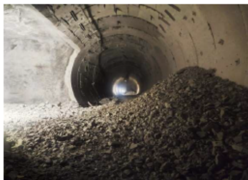
Excavation of Adit from Tunnel I to II for manual excavation in Tunnel II. Until closure of Adit, release of water through tunnel I is not possible
