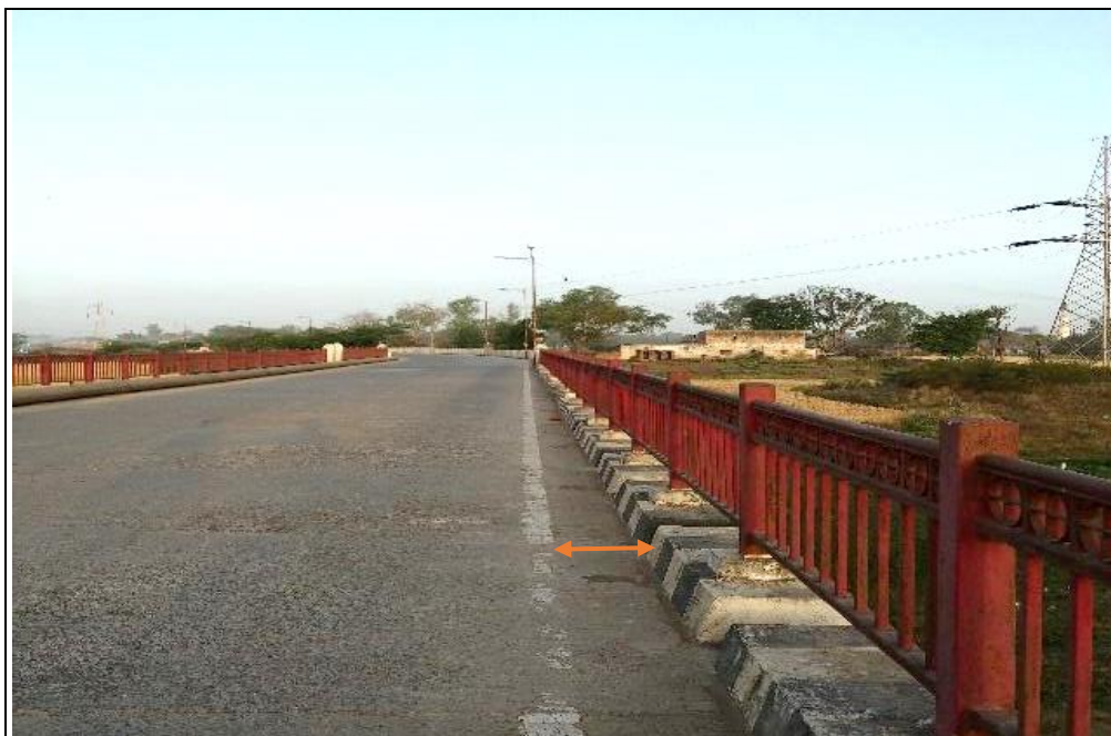
Submersible Bridge on Rinmukteshwar to Ranjeet Hanuman Road (Ujjain) with insufficient kerb width.
