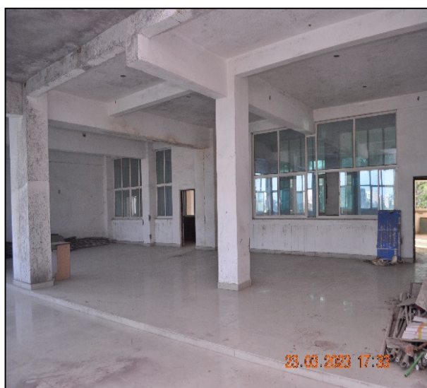
Picture No. 2.1: Incomplete structure on 2 nd floor of existing Block-A
