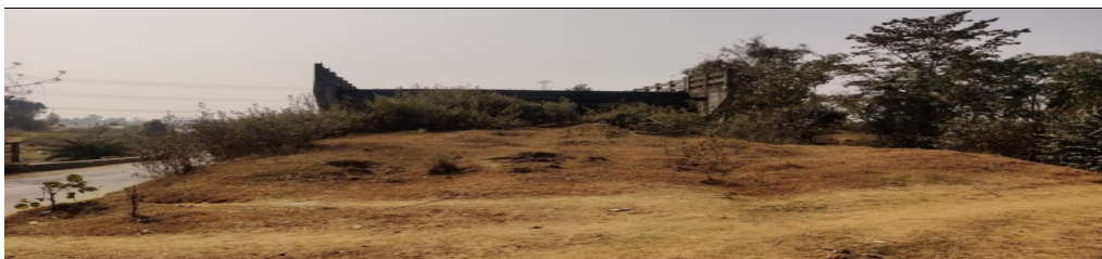
Photograph of the idle bridge (January 2021)
