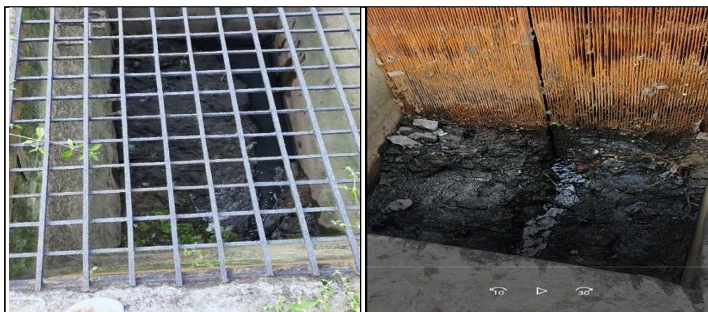
Picture 4.7: Chamber before STP-5 and the screen chamber of STP-5, filled with solid deposits
