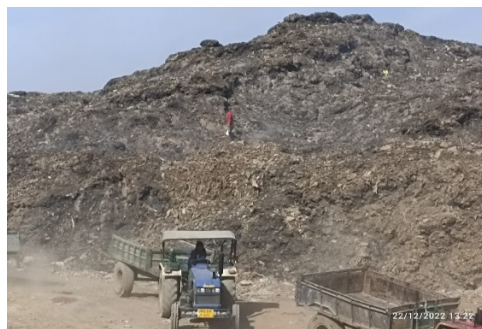
Municipal waste dumping site at Jhiri, Ranchi.
