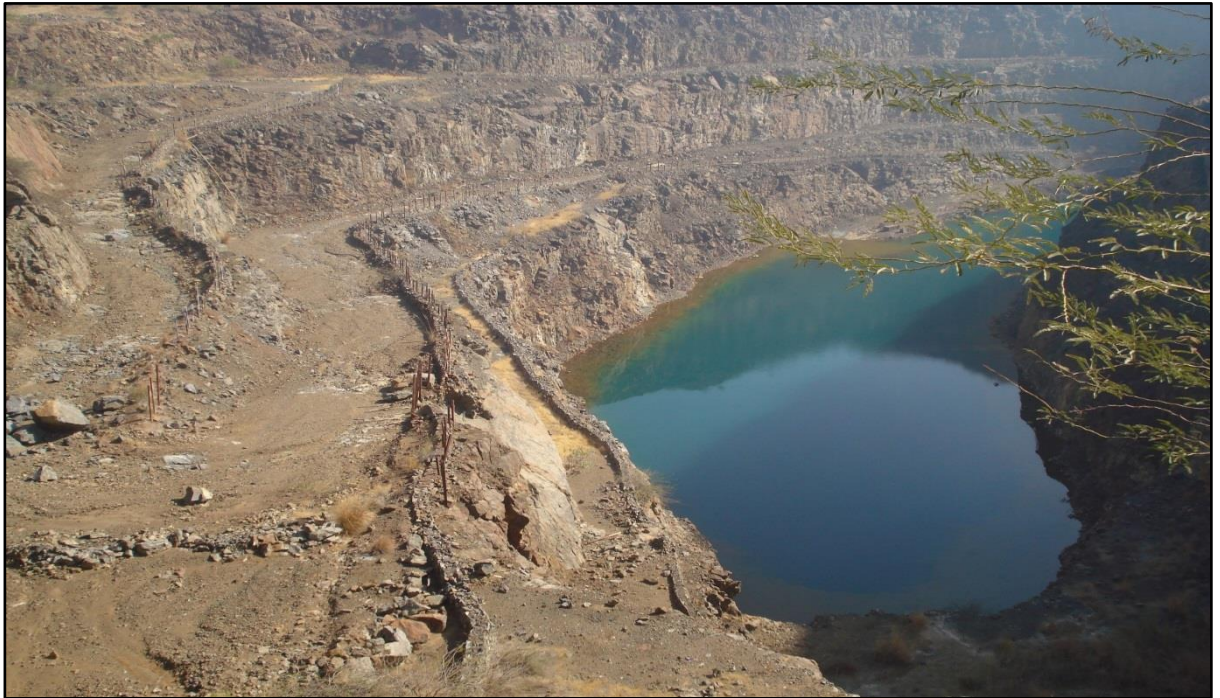
Figure 3.2: Benches of Chandmari open cast mines
