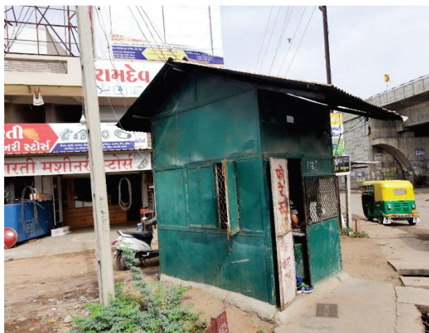
Photograph 5.1: Naka on Deesa-Palanpur Highway Photograph taken by Audit on 21 July 2021
