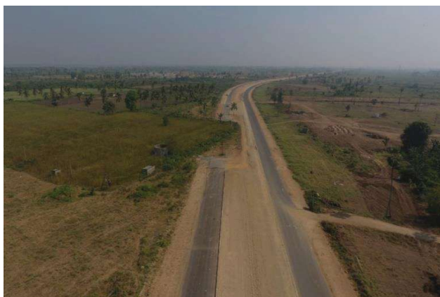
Picture 4: Showing construction of additional lanes on SAR
