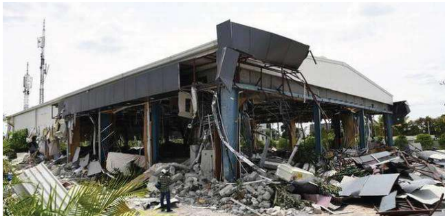
Picture 6: The demolished Grievance Hall as on 26 June 2019
