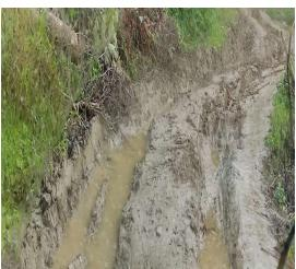
Pic: Link-road without side drain and gravel
