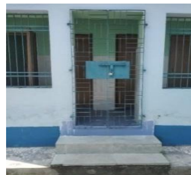
Picture 2.6: Toilets of Workshop, Govt. ITI, Malda
