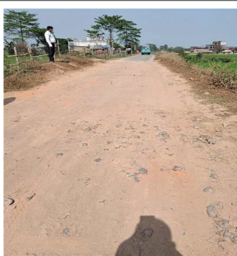
Fig. 2.16: Uncovered non-bituminous layers
