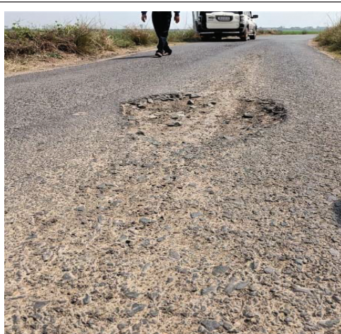
Fig. 2.15: Potholes generated
