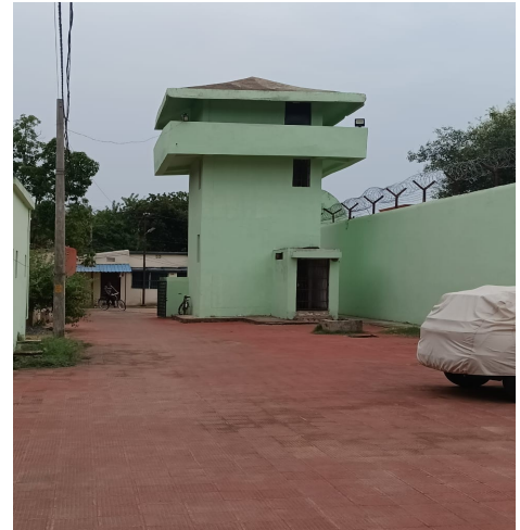
Photo No. 11: Watch tower without any personnel or security equipment, Special Jail, Bhubaneswar
