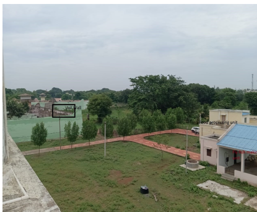
Photo No. 12: Idle food processing unit at Circle jail, Berhampur
