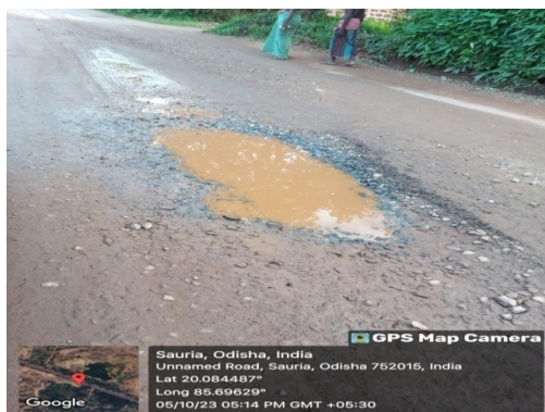
Photo No-6: Non-executed portion of Pattanaikia-Delang-Khordha road with big potholes (Khordha R&B)
