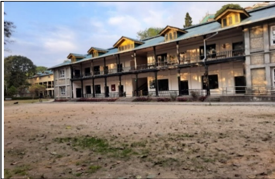
Image 3: Lid of chambers buried 0.50 to 1.00 foot beneath the playground, PNG School
