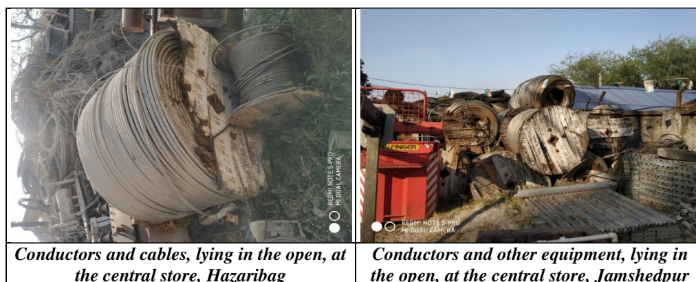
Picture 5.1: Pictures of material kept haphazardly in CSs
