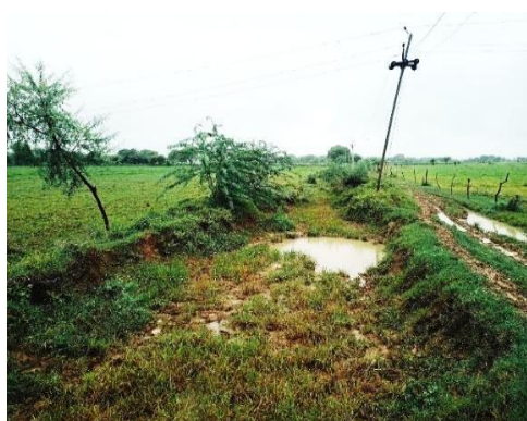
Field channel not constructed at Italia Minor (DCS)
