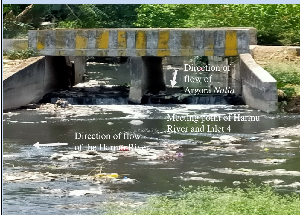
Picture 4.5: Discharge of sewage directly, through Inlet 4, into the Harmu river
