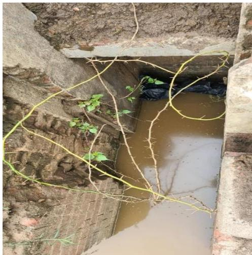
Regulator gate not installed at the head of Masoodpura minor of DCS
