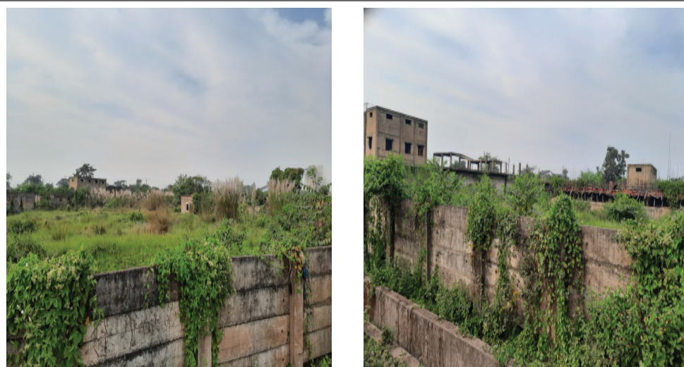
Fig. 2.18 and Fig. 2.19: Abandoned site in dilapidated condition (December 2021)
