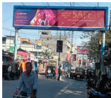
Fig.2.15: Overhead hoarding installed blocking shoulder and footpath area at junction of Suniti Road and Keshob Road under Cooch Behar PW Division (01.01.2021)
