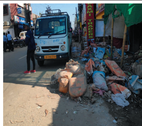
Fig.2.9: NN Road at 0.400 km (01.01.2021)
