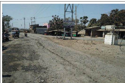
Fig.2.13: Intersection at 2.7 km on Nalhati Bhabanandapur Road under Birbhum Highway Division-I (27.02.2021)
