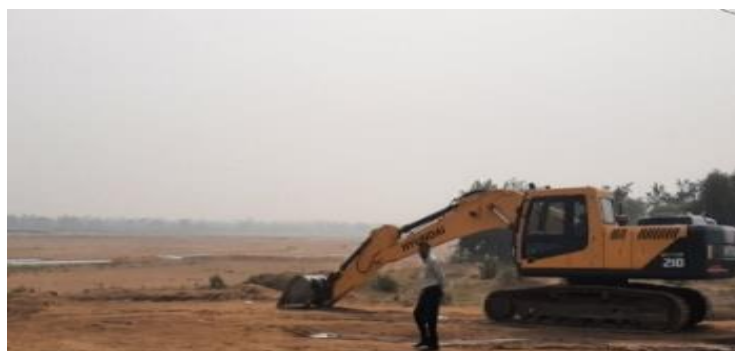
Figure- 4.2: Use of Poclain machines at sites (Balodabazar District, date of image: January 2021)
