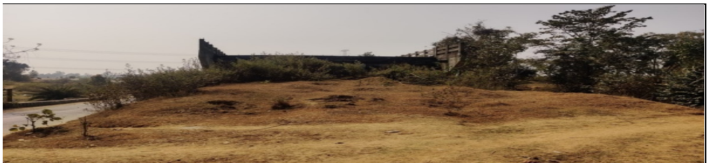
Photograph of the idle bridge (January 2021)
