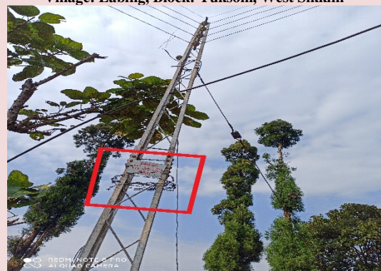
Lesser quantity of barbed wire used Village: Ringhim, Block: Mangan, Dist: North Sikkim
