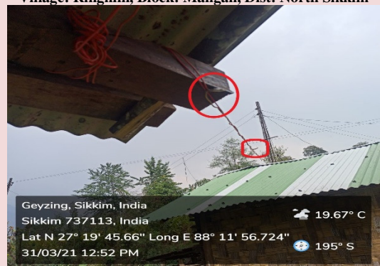
Internal wiring cable knotted with the service cable due to short supply of 2.5 mm service cable Village: Chojo, Block: Yuksom, West Sikkim
