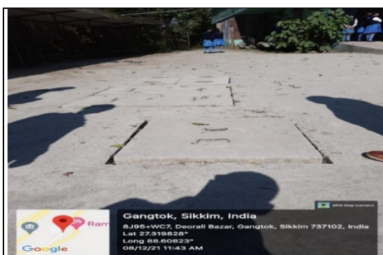
Image 1: Closure lids of chambers not as per specification Deorali Girls High School
