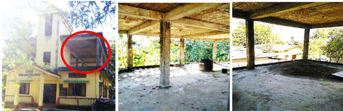
Incomplete 1 st floor of the Block Resource Centre under Katlichera AP
