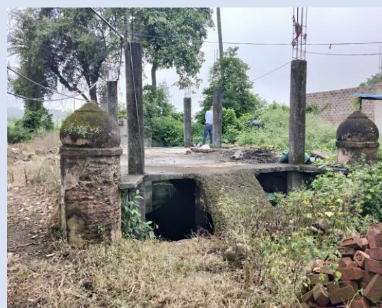
Picture 3.23: Concrete slab and columns were noticed over Prachin Bawri No.1, Choti Jam, Mahu, Indore (23-09-2021)
