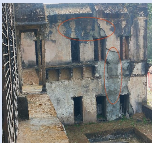
Picture 3.46: Cement used in repairing of wall of Moti Mahal, Ramnagar, Mandla (07-12-2021)
