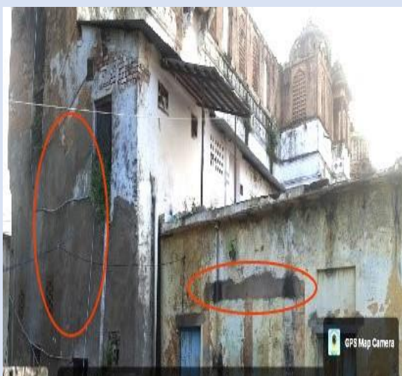
Picture 3.47: Cement used in plastering of wall at Jujhar Singh Mahal, Orchha (23-09-2021)
