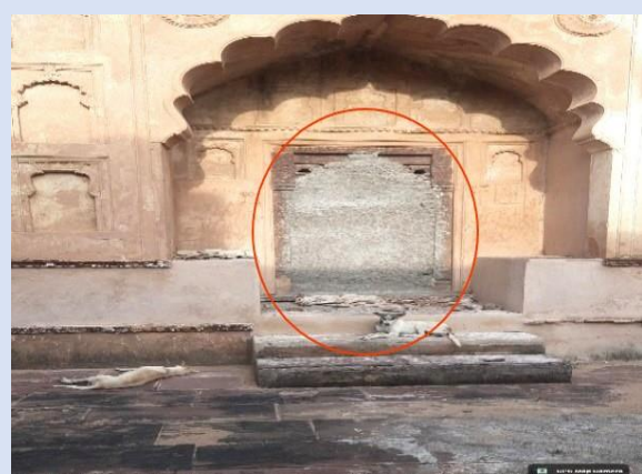
Picture 3.48: Cement used to close the entrance of Raiman Dau Ki Kothi at Orchha (24-09-2021)
