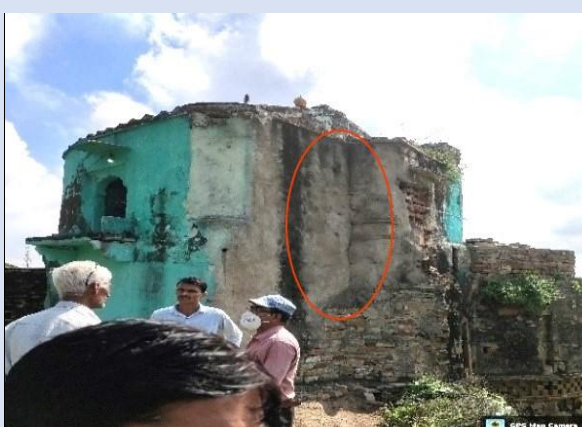
Picture 3.49: Cement used in repairing work of wall of Garhi Sumawali, Morena (14-09-2021)
