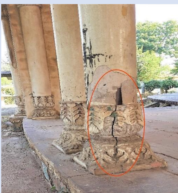
Picture 4.29: Deteriorated pillars of District Museum, Rewa (22-11-2021)
