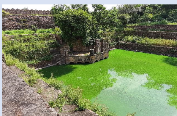
Picture 3.40 and 3.41: Vegetation on the walls of fort and growth of algae in Suraj Kund, Hinglajgarh Fort, Mandsaur (07-10-2021)
