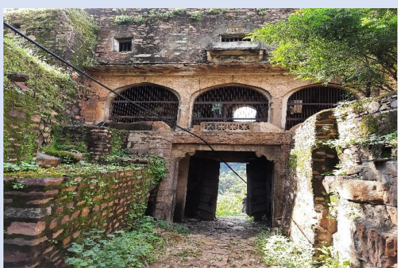
Picture 3.40 and 3.41: Vegetation on the walls of fort and growth of algae in Suraj Kund, Hinglajgarh Fort, Mandsaur (07-10-2021)
