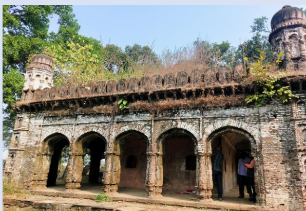
Picture 3.39: Vegetation on the roof of Aasaf Khan ka Maqbara, Mandla (07-12-2021)
