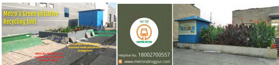
Figure 3.8: Bio Digester installed at Airport South Station
