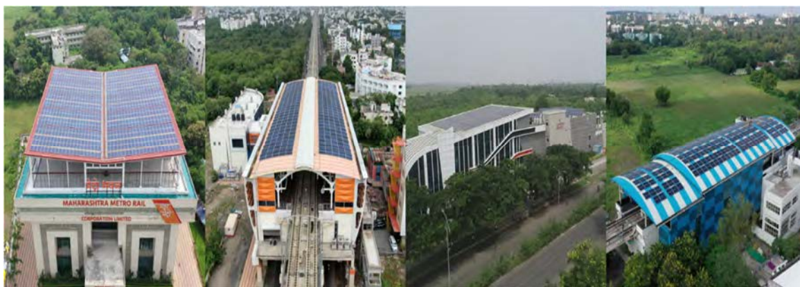
Figure 3.7: Roof top solar panels at Metro Bhawan and metro stations
