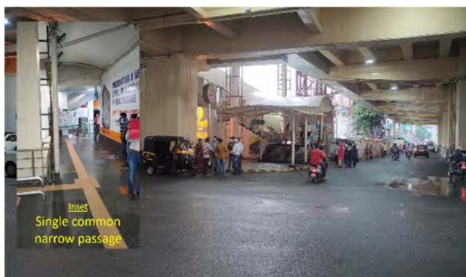
Figure 3.5: Single entry/ exit at Sitabuldi Station
