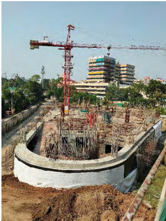
Figure 5.1: Construction of two level parking facility at Kasturchand Park
