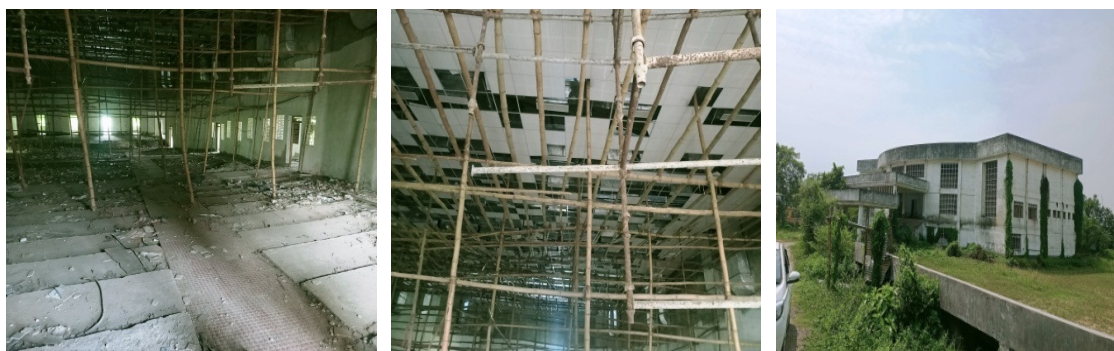
Photographs 2.5.1, 2.5.2 and 2.5.3: Status of construction of Auditorium
