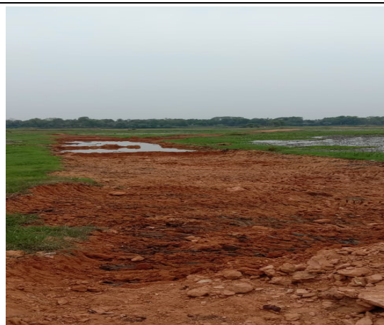
Photograph 3.6.5: Rajghat to Yubarajghat (during removal of earth)
