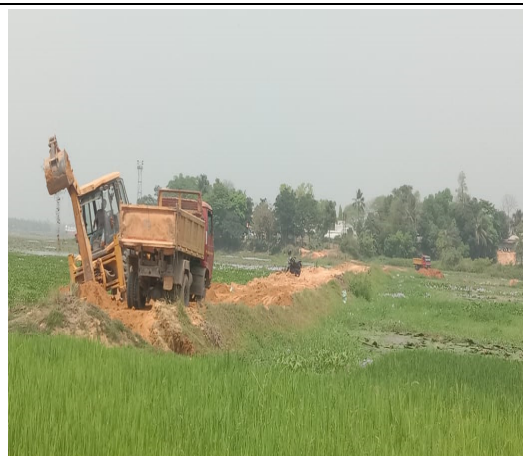
Photograph 3.6.4: Rajghat to Pacharmarghat (during removal of earth)
