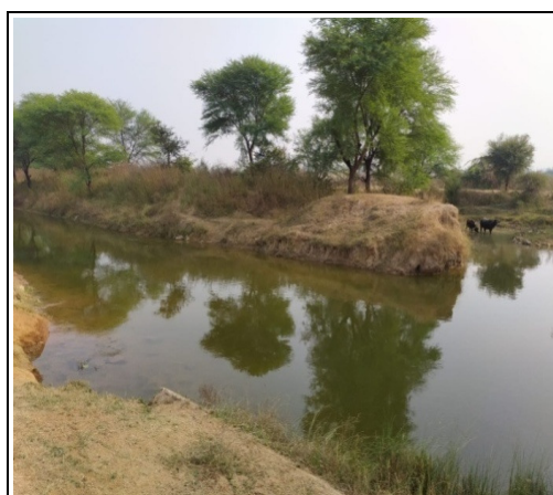
View of breach of Right Bank Canal (Up to Mahuar river) before Samoha pickup weir. (Status: December 2019)
