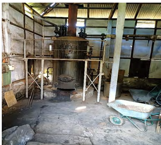
Condition of existing FPU
