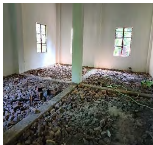
Incomplete New FPU
