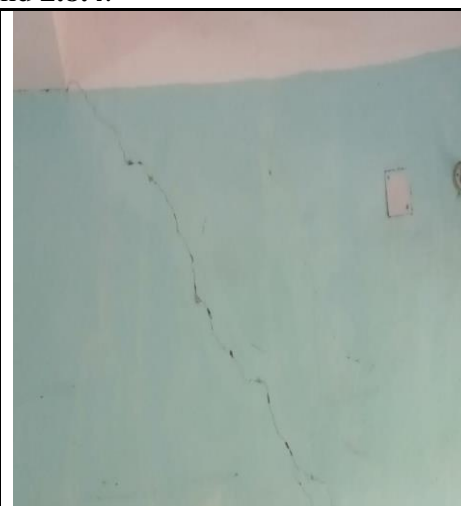
Picture 2.8.4: Diagonal cracks on the walls (30.06.2022)
