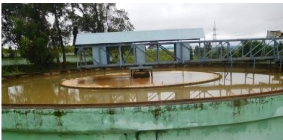
Picture 2.3.7: Non-functional trolley and high turbid water in Water Treatment Plant at Sunabeda (27.07.2023)
