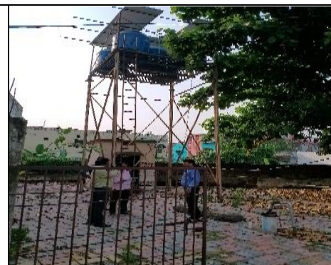
Picture 2.3.6: Defunct solar project at Baikuntha Nagar, where one solar panel and motor pump was missing (05.09.2023)
