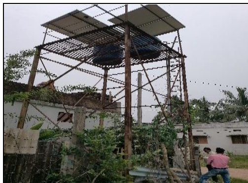
Picture 2.3.5: Defunct solar project at Nua Sahi, Ankuli, where some solar panels and three water tanks were missing (05.09.2023)
