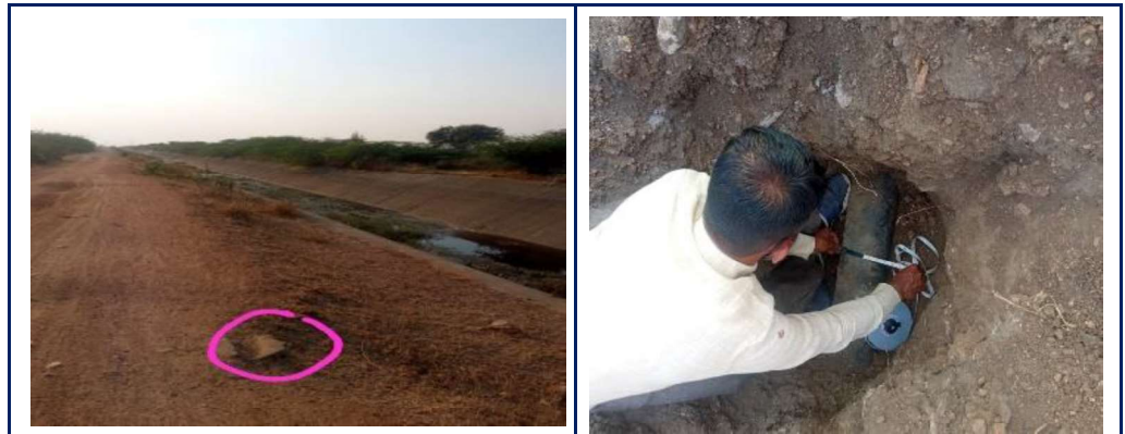
Exhibit 4.11: Incomplete pipeline work
