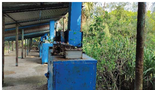
Fig. 35: Rusted dryers left unused at Purunabandha
