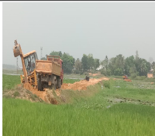
Photograph 3.6.4: Rajghat to Pacharmarghat (during removal of earth)
