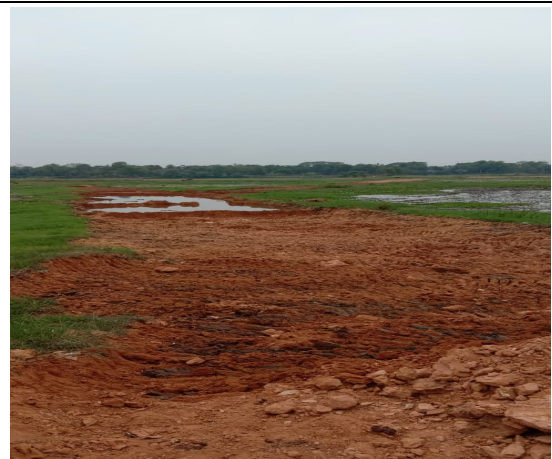
Photograph 3.6.5: Rajghat to Yubarajghat (during removal of earth)
