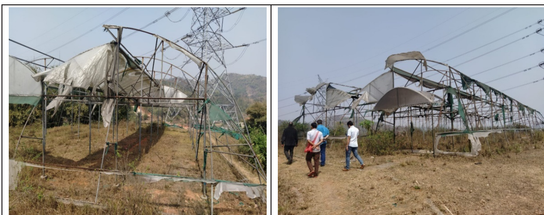
Fifth Green House in front of the office building and below the labour barrack was found in a dilapidated condition. No plantation was observed under the green house (12-03-2021)
