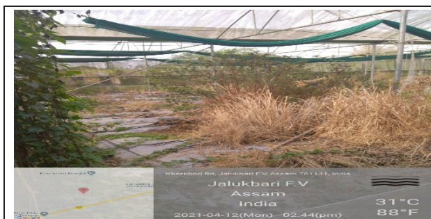
Green house (stated for root stock) roof damaged and full of bushes (12-04-2021)
