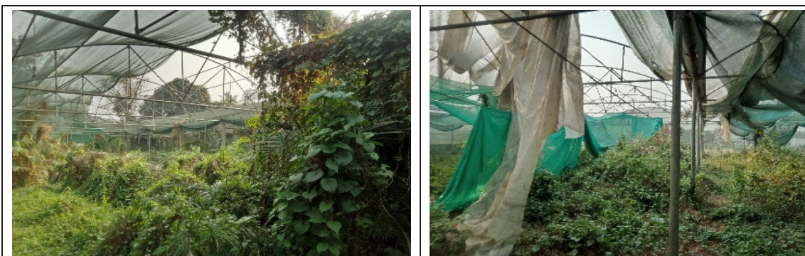
Green house in damaged condition full of jungles and bushes. Shade net of roof and side wall also missing at places (24-03-2021)
