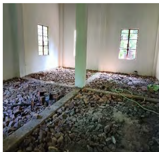
Incomplete New FPU
