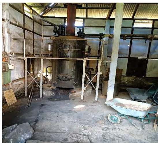
Condition of existing FPU
