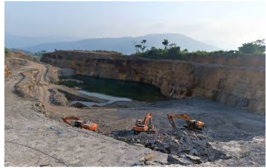
No gullies/drainages provided in the mining lease site at Lumshnong area under DFO(T), Jowai
