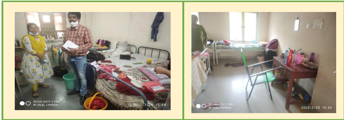
Figure 5.3 - Inadequate space and furniture in Girls Hostel of OMC (29 March 2022)
