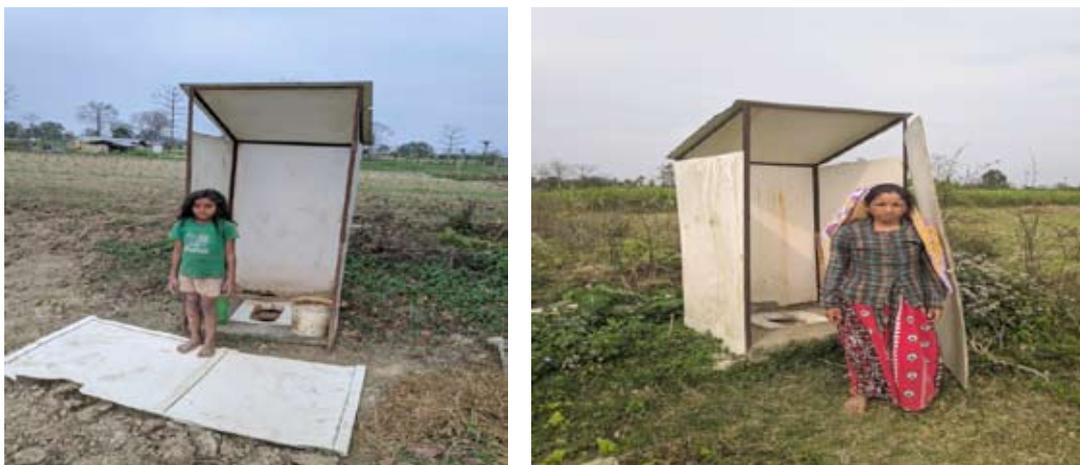
*Dilapidated condition of the pre-fabricated toilets*
