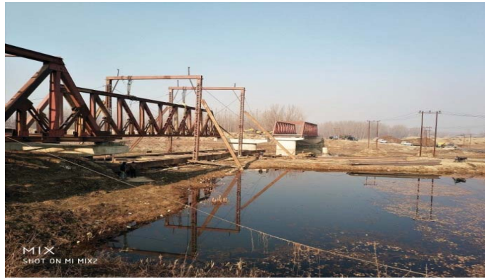
(Incomplete bridge over the FSC at Shariefabad 28 December 2019)
