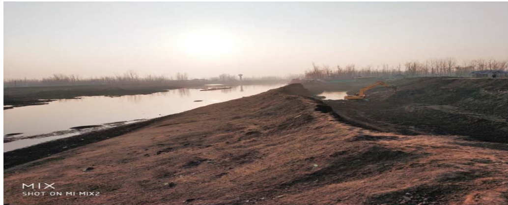
Picture showing unexcavated portion of FSC at RD 38.068-39.860 on 28 December 2019
