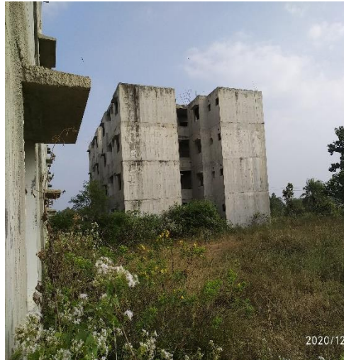
Partial super structure 1BHK block
