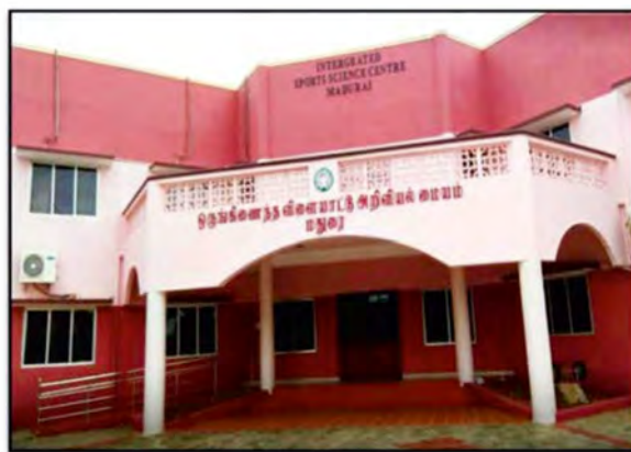
Exhibit 3.1 : Integrated Sports Science Centre, Madurai
