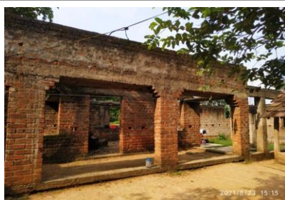
Incomplete Kitchen-cum- dining room at CCI, Mangalpur
