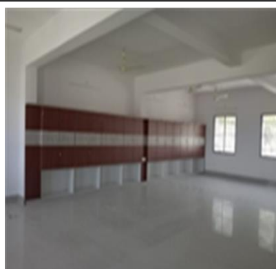
Inside view of the newly constructed CCI at Bhawanipatna
