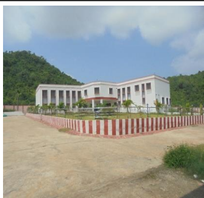
Newly constructed CCI at Bhawanipatna
