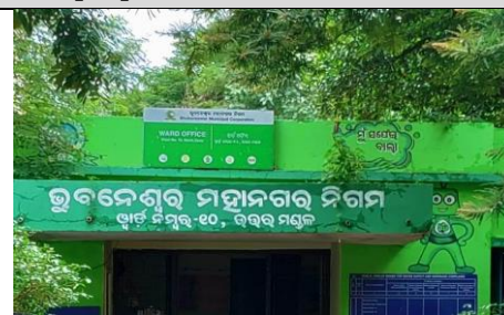
WWH at Mancheswar is used as BMC Office, Ward No.10, Northern Circle
