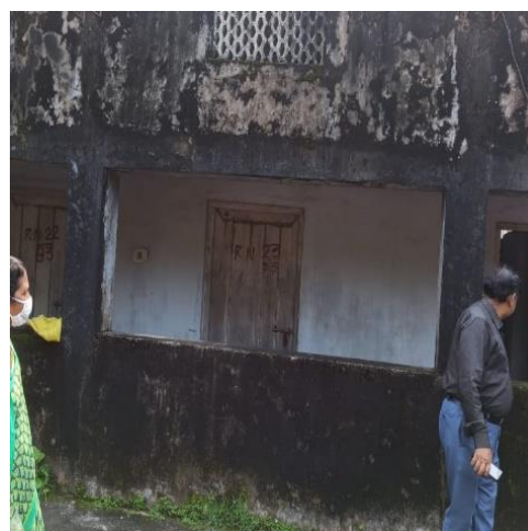
Outer condition of the first floor
