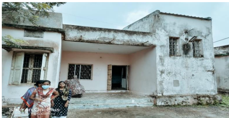
WWH at Bhanjavihar in dilapidated condition
